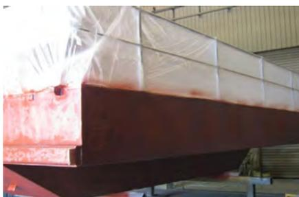
**2** BLASTED SUBSTRATE coated with **Erabond 6100FC Red** primer. This is a fast cure priming system with an added anti-corrosive package.
