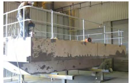
**1** PONTON SURFACE PREPARATION consisting of 2½ class blast of new steel and repaired steel sections and whip blast of existing paint sections. Substrate washed with solvent after blasting.
