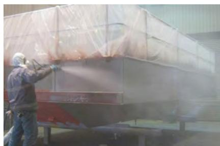
**3** SPRAY APPLICATION to 3mm coating thickness of **Eraspray ESM900 grey** via high pressure impingement mixing equipment.
